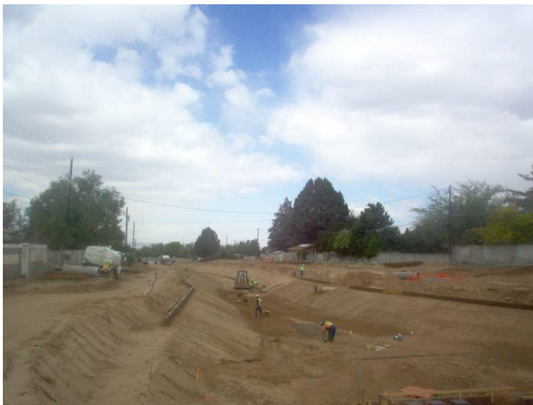
PRS placing rebar west of the WQS. RMCI placing top forms.
