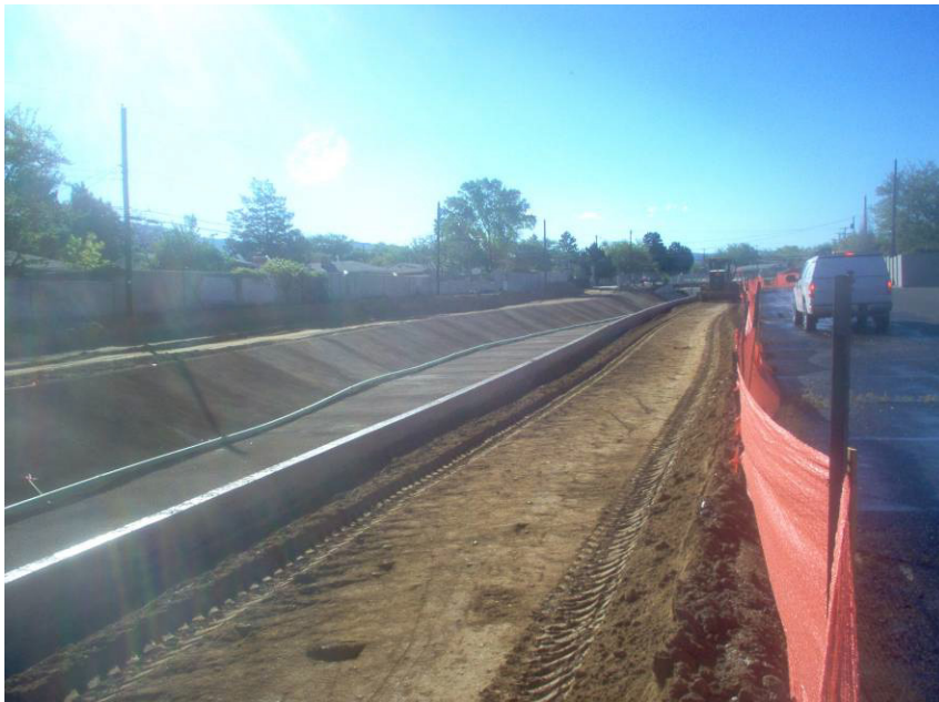
Guzman bring up lifts on the south side of the channel.
