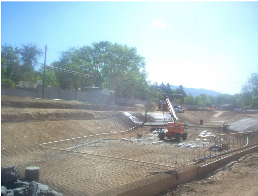
Superior placing shotcrete at upper end of the WQS.
