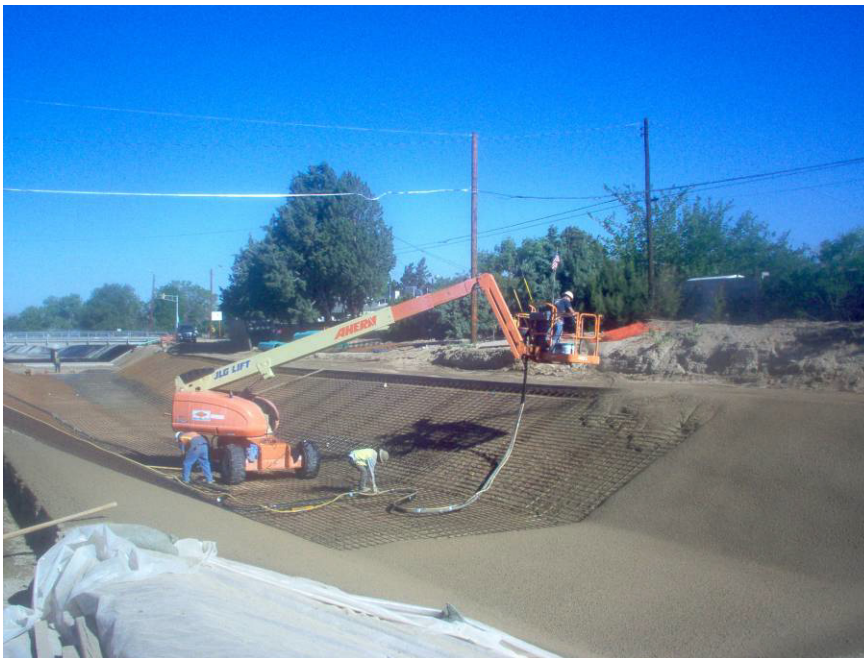
Superior placing shotcrete.
