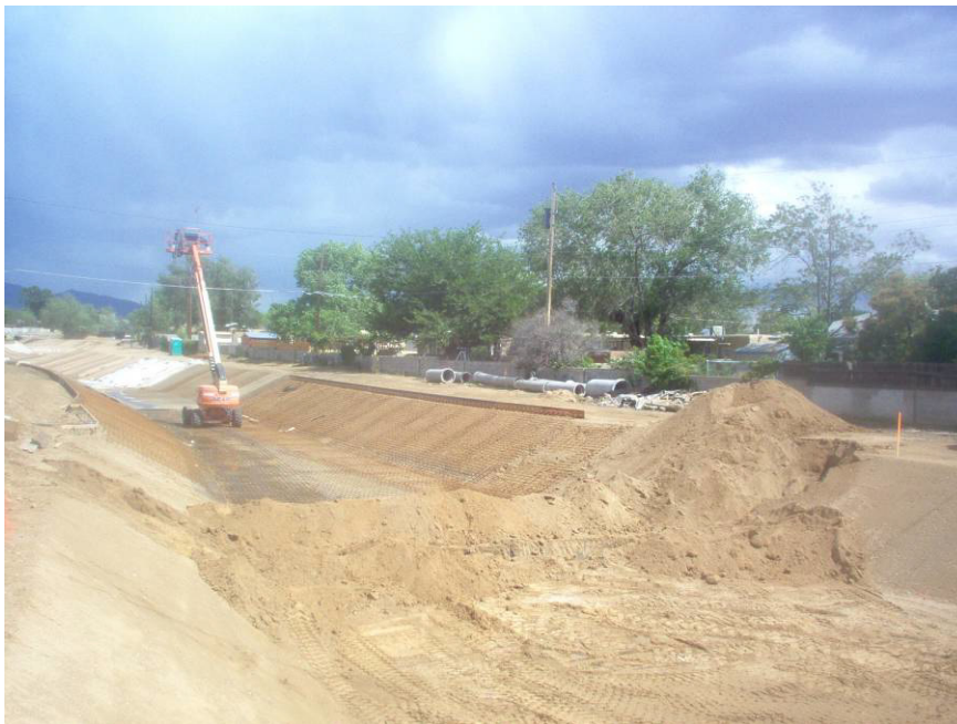
RMCI trenched for irrigation crossing at 6+25.
