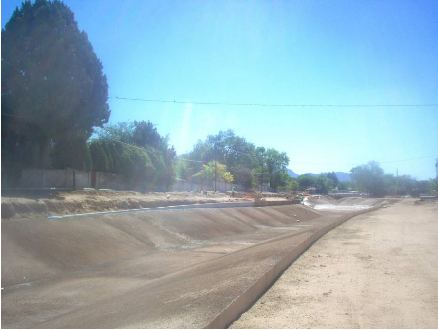
Contractor cleaning and rubbing sill wall. 11+00 to 12+50
