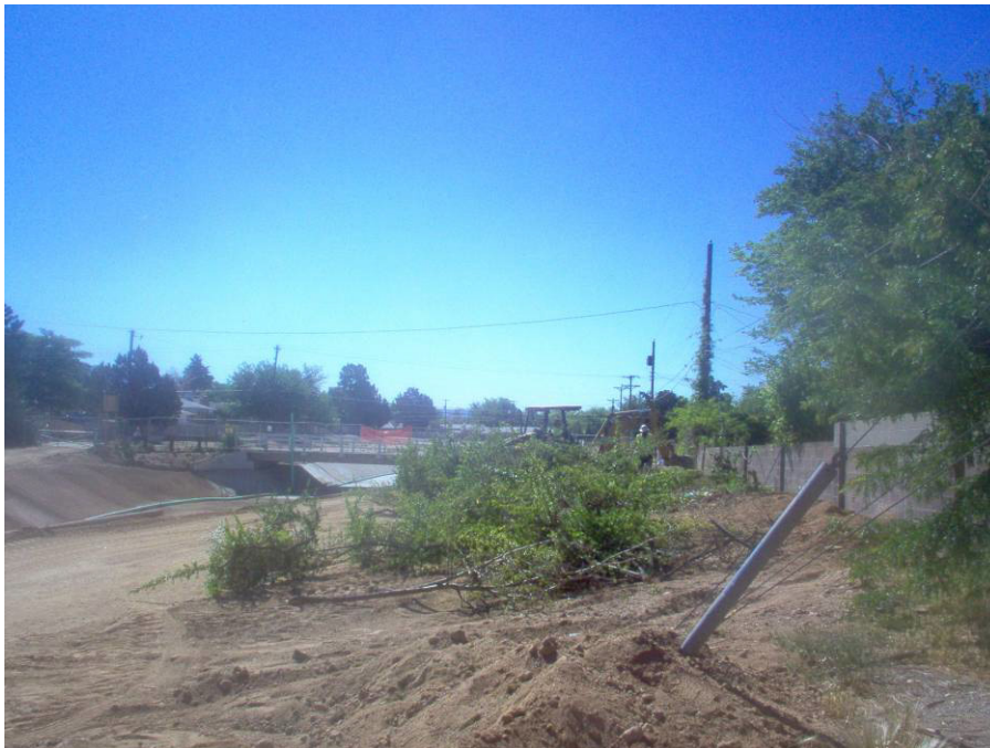
Guzman removing vegetation inside the right of way.
