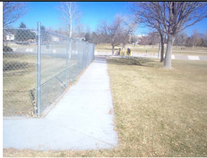
Sidewalk that runs along the east side of the Senior Center
