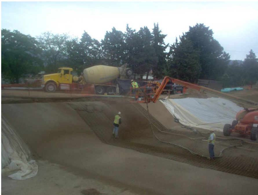
Superior placing shotcrete tying into the existing channel at the BOP.
