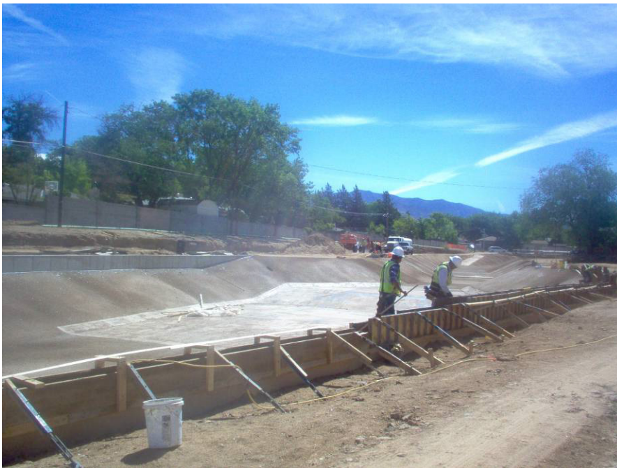
RMCI forming sill wall on the south side.
