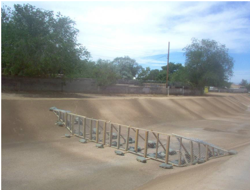
Temporary WQS placed west of the San Pedro Bridge.
