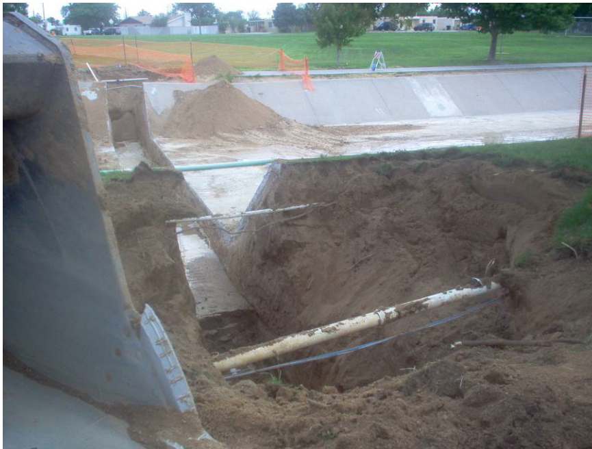
At irrigation crossing 4" waterline encountered and will be repaired today.
