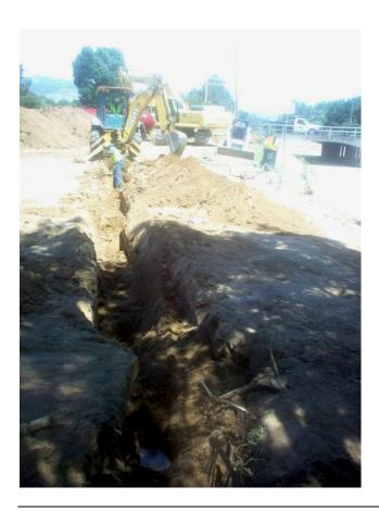
RMCI relocating existing 4" irrigation line north side of the channel.
