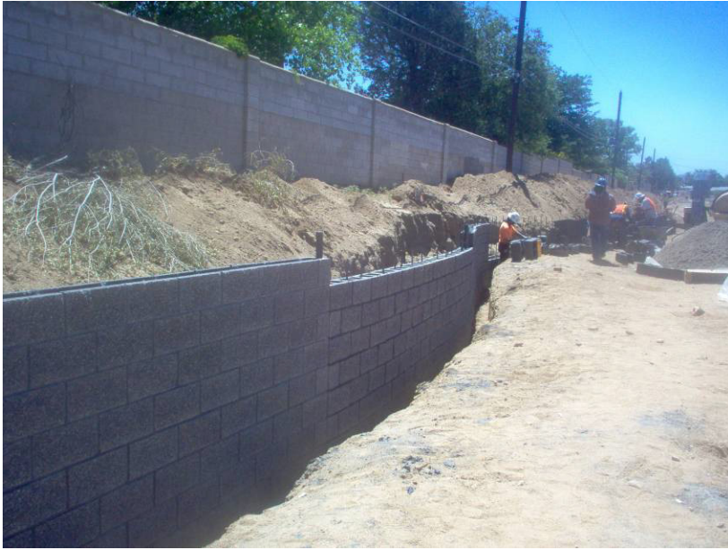
Peerless (Indian Investors) placing block wall.
