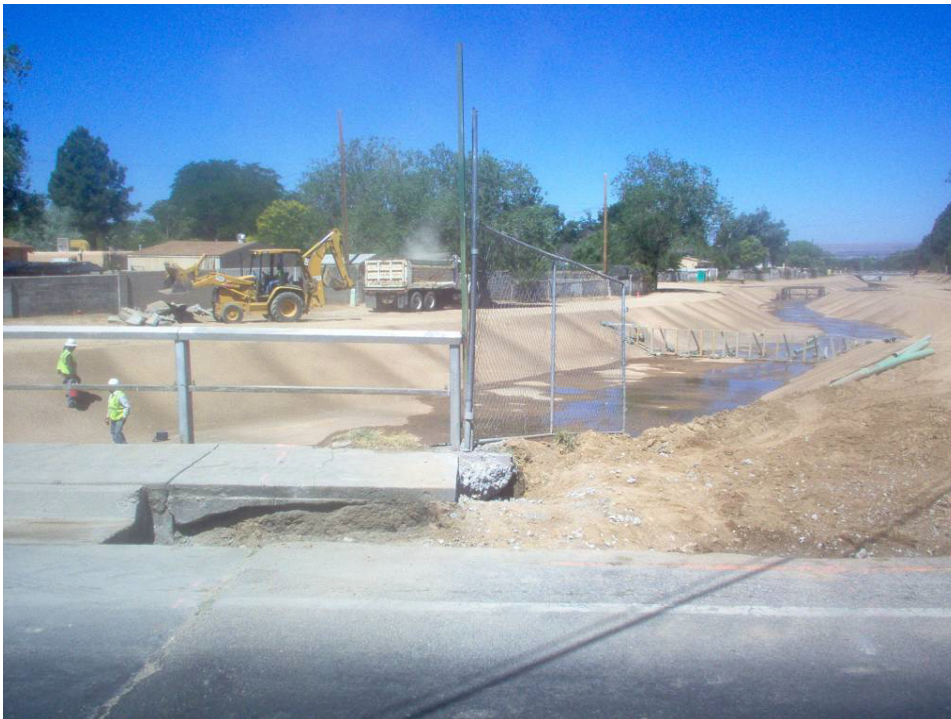
Guzman hauling off concrete removal debris from site.
