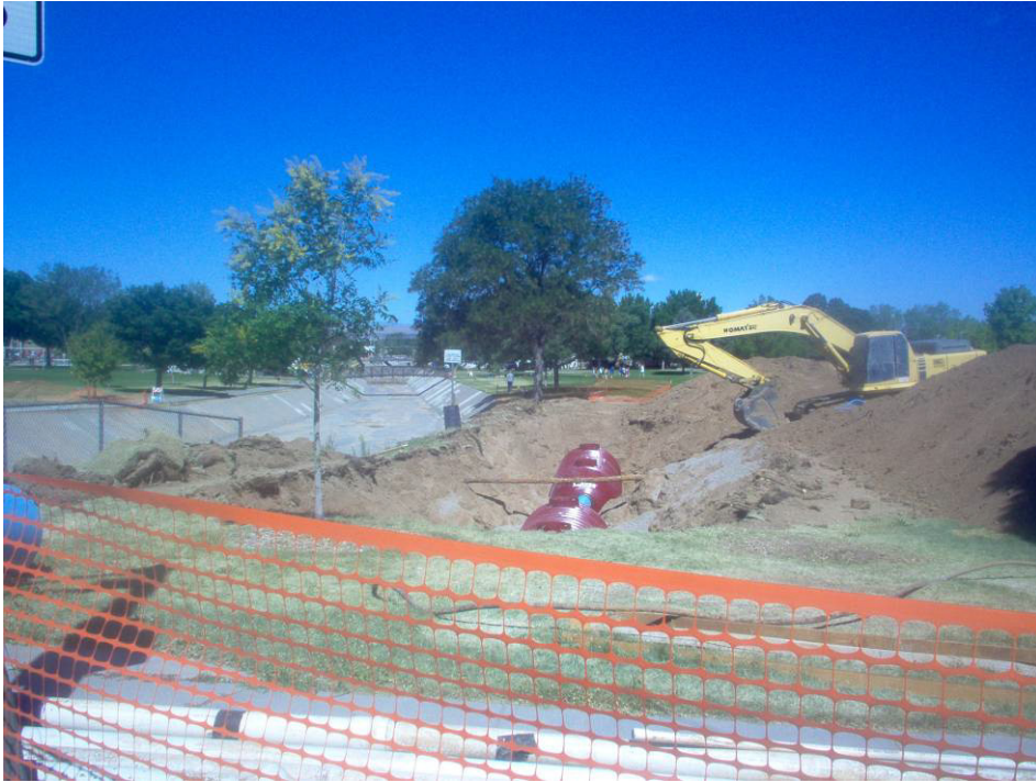
RMCI placing the fiberglass tanks for the Water Harvesting.
