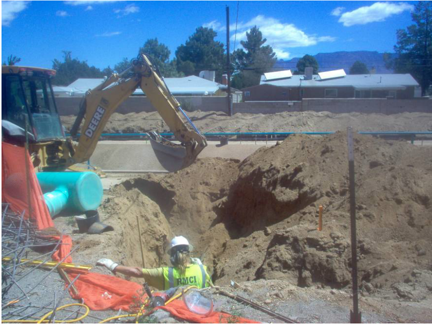
RMCI placing area drain at Sta 26+79
