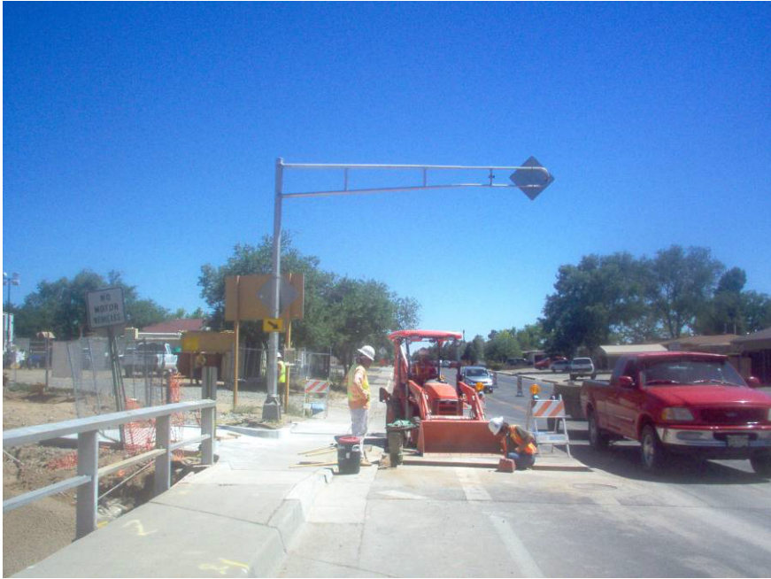
Land- Tek placing sleeves across San Pedro within barricading.
