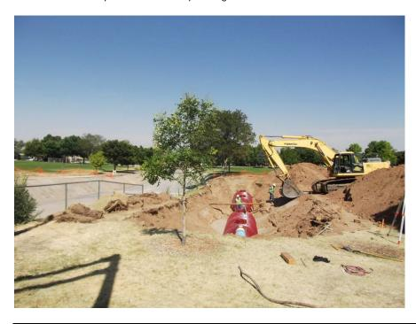
RMCI re-adjusted the tanks, placing new gravel and will begin compaction.
