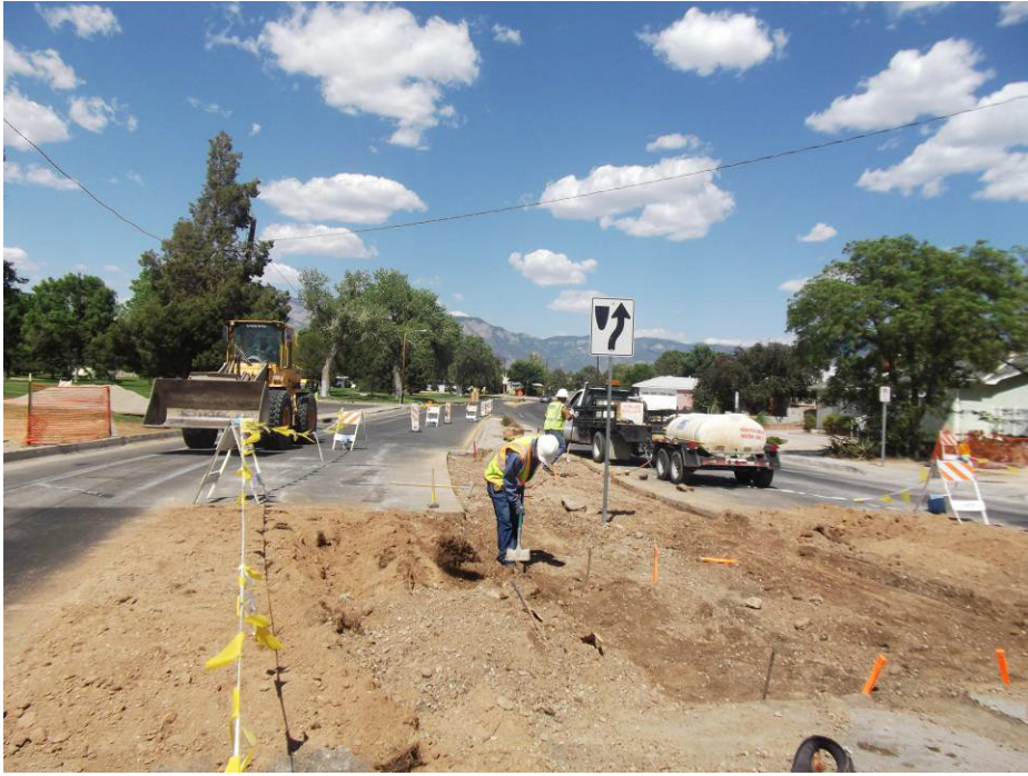
HO preparing to place median curb and gutter on Comanche.
