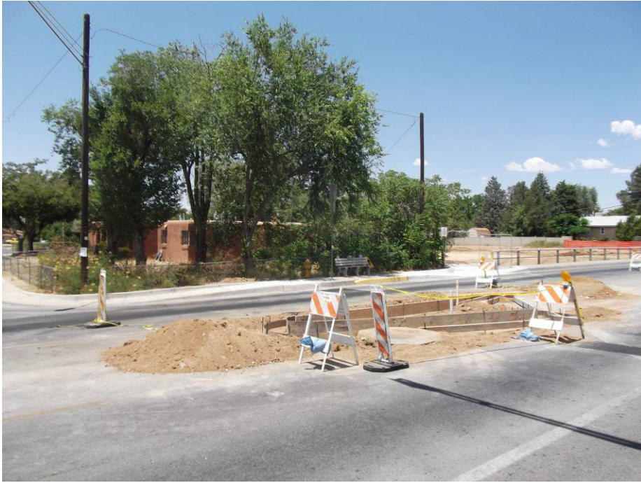
HO preparing to place median curb and gutter at San Pedro.
