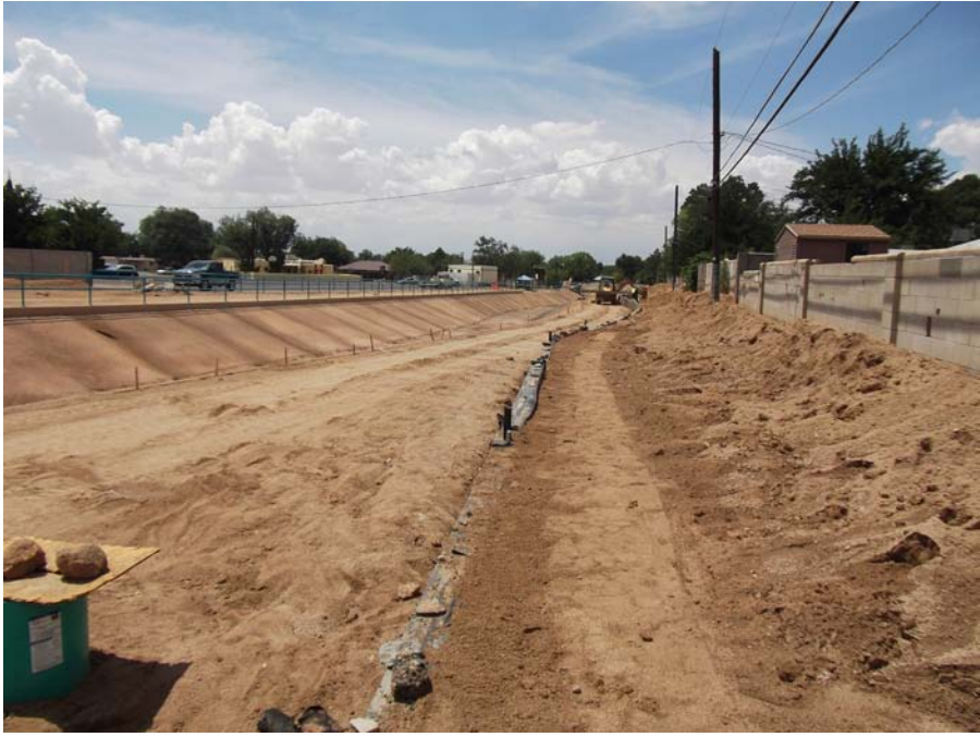
Peerless compacting behind Wall "C"
