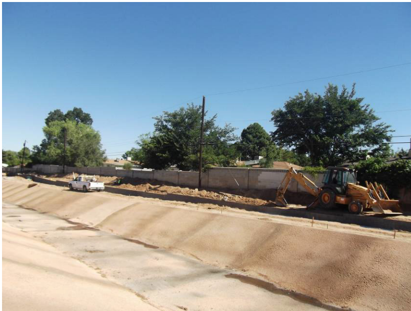
Peerless digging footing for Wall "D"
