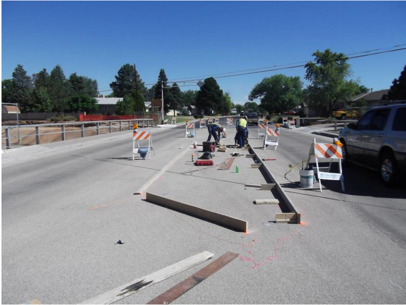
HO setting forms for pin curb in San Pedro
