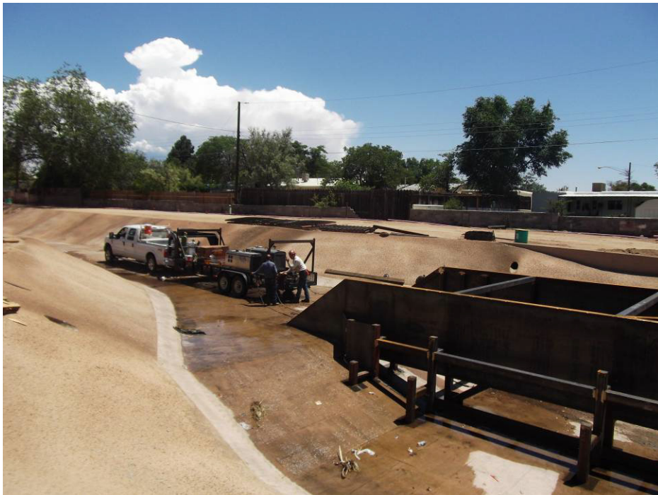
D&R Tank Welders at WQS
