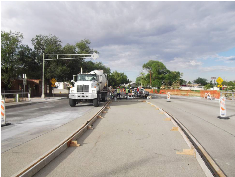
HO Pouring pin curb on Comanche
