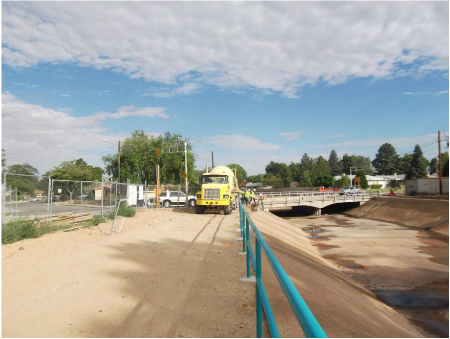
RMCI pouring sill walls at San Pedro
