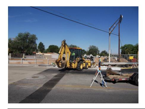
HO removing and replacing the DW at the NW quad of the San Pedro Bridge
