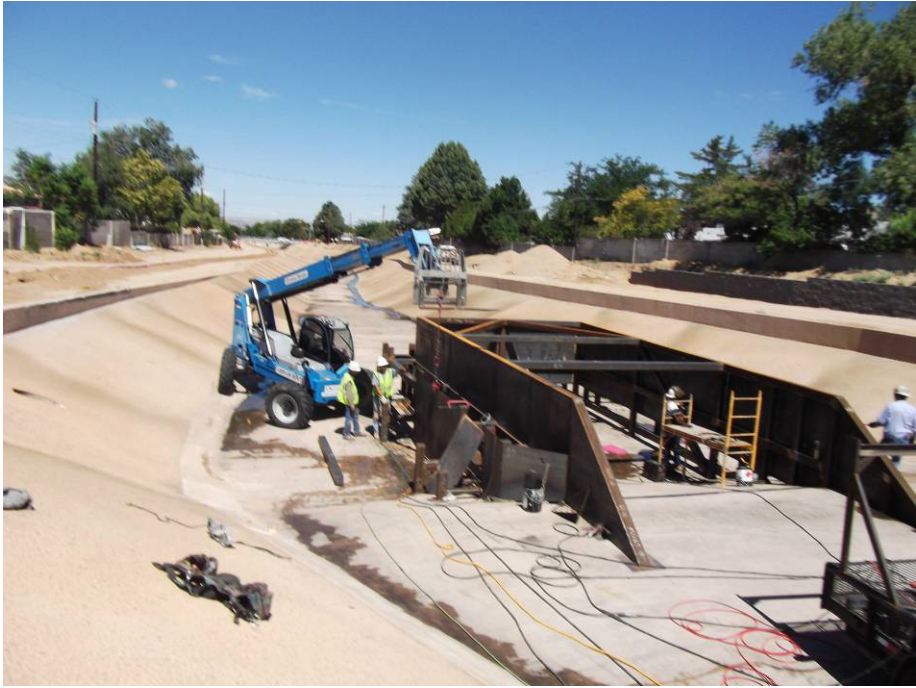
D&R Tank and RMCI continues to place skirt at WQS
