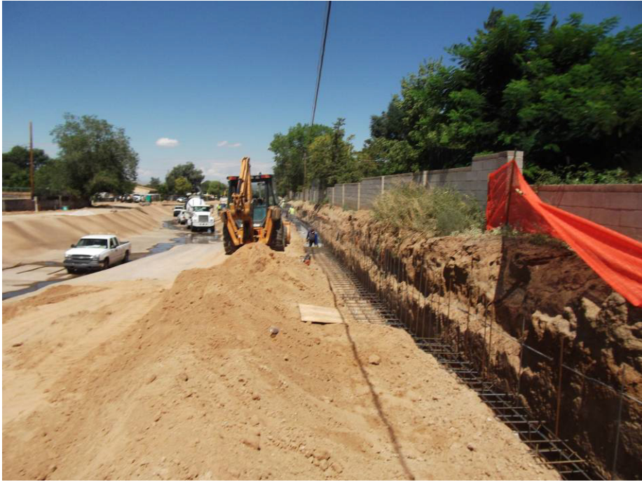
L footing on "B" wall poured today at 1:00 pm
