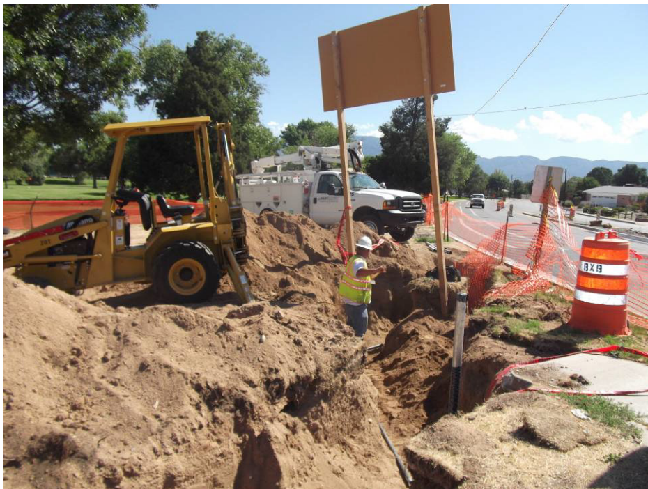
Bixby placing rigid conduit to power riser.
