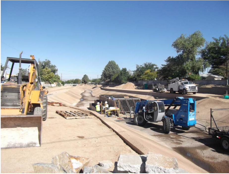
D&R tank and RMCI working the finishing touches on the WQS
