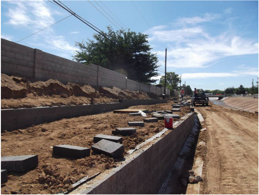
Peerless laying out cap block for walls "C" and "D"
