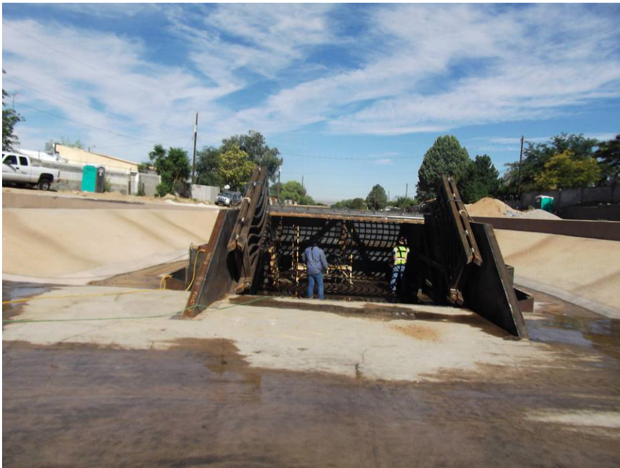
JD Inspection and a welder from RMCI going over punchlist items.
