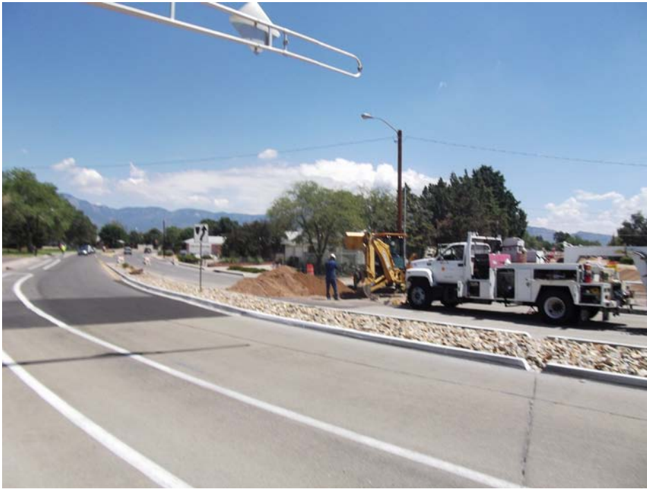
Gas Co of NM capping gas service under Comanche.
