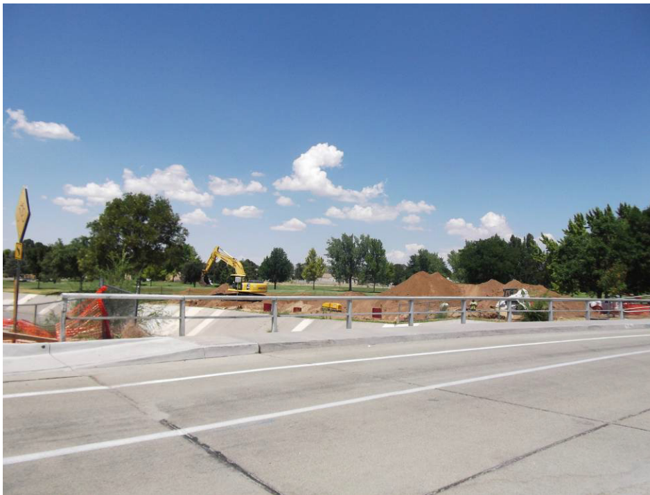
RMCI digging for water booster station west of Comanche
