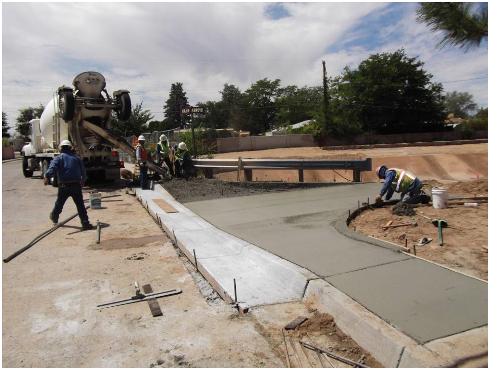
HO pouring the driveway at the NW quad of California Bridge.
