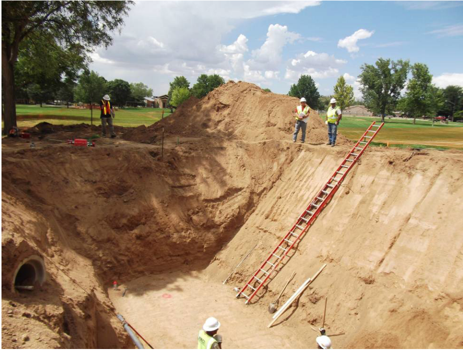
Trench being prepared for forms and rebar will pour tomorrow.
