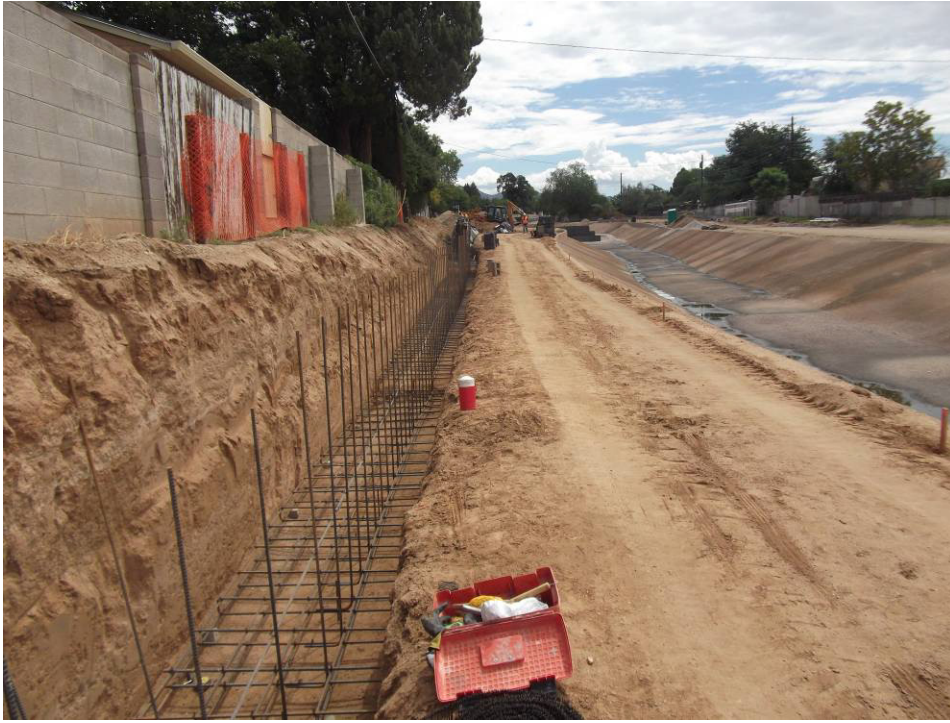
Peerless placing rebar in footing and then poured at 1:00 pm
