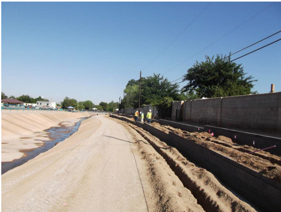
Land Tek cleaning trench for placement of irrigation main.
