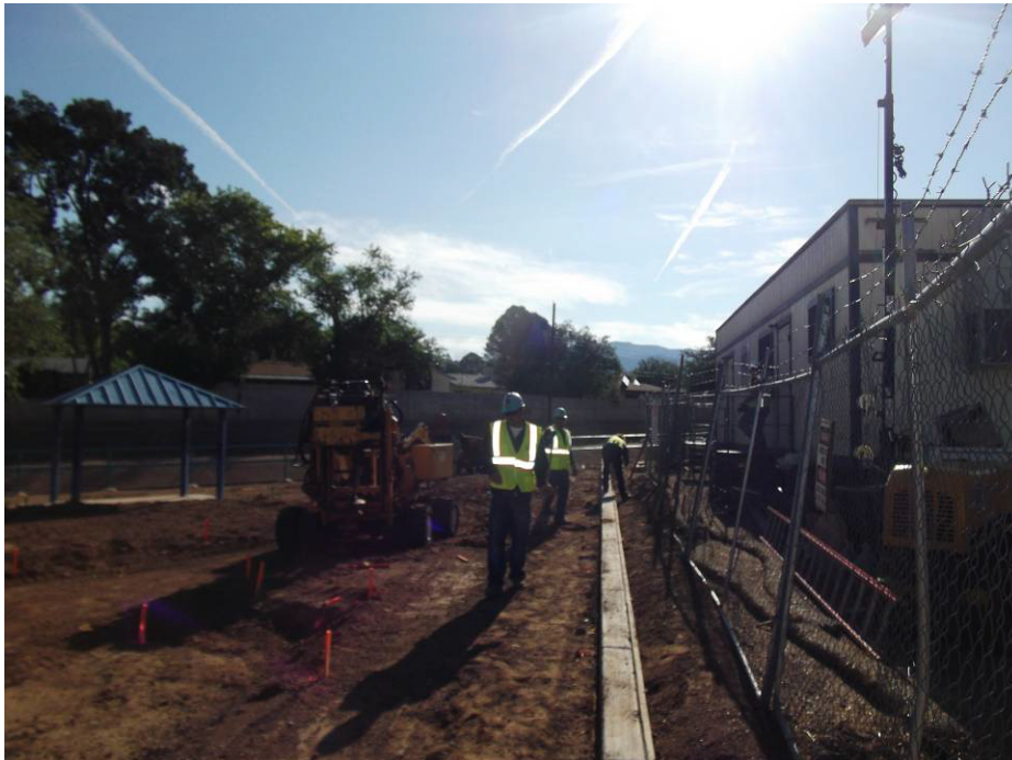
Scotts Fence drilling holes for verticals on pipe rail fence.
