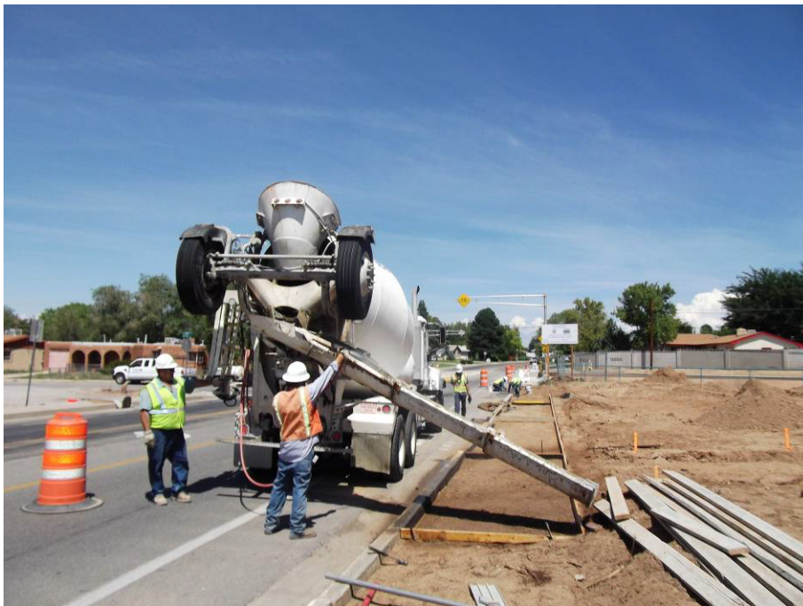
HO pouring back sidewalk on San Pedro
