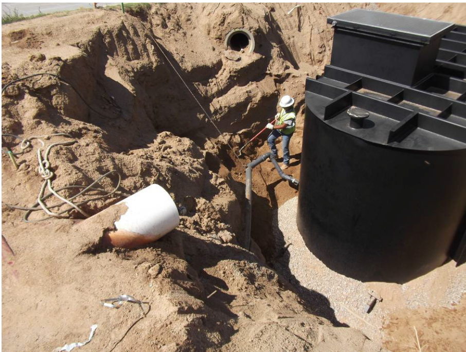
Water Booster Station. RMCI placing gravel.
