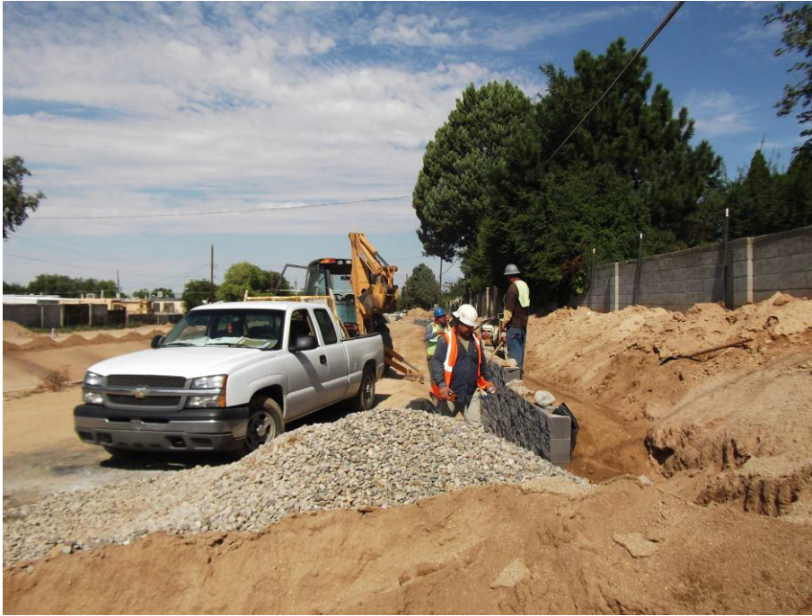
Peerless backfilling behind Wall “A”.
