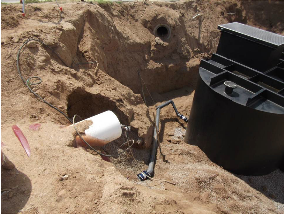
RMCI changed out the couplings to the higher rated couplings that Smith requested.
