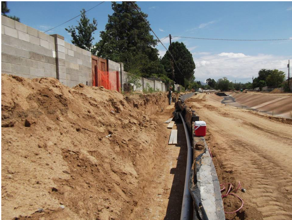
Peerless continues to place drain line and backfill on wall "A"
