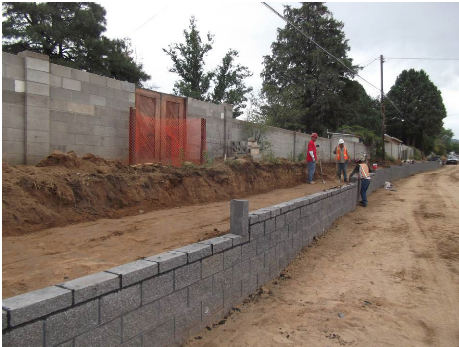
Peerless placing cap blocks and backfilling behind wall "A"
