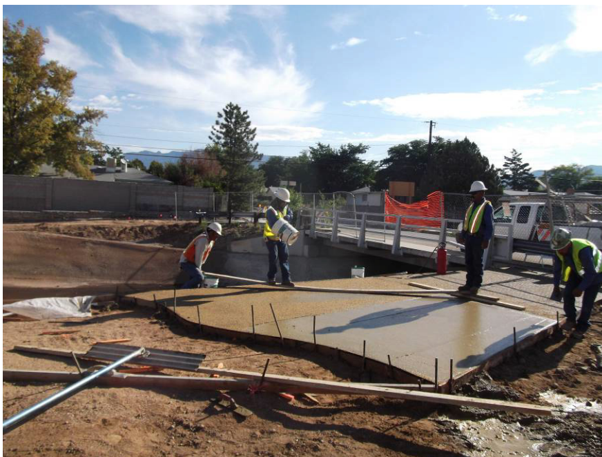
HO placing exposed aggregate concrete on plaza NO. 7.
