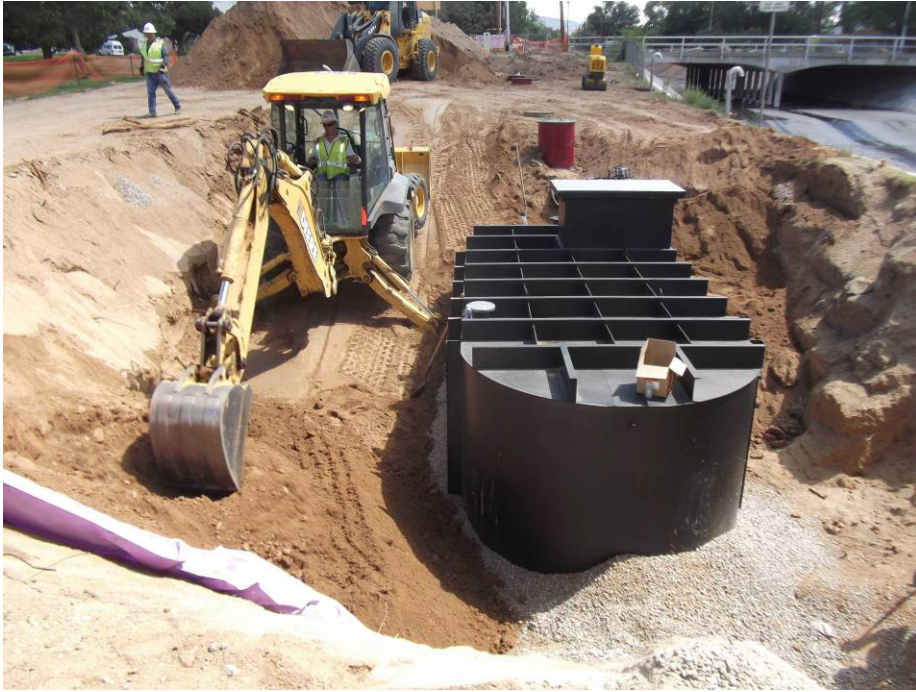
RMCI backfilling around the water booster station.
