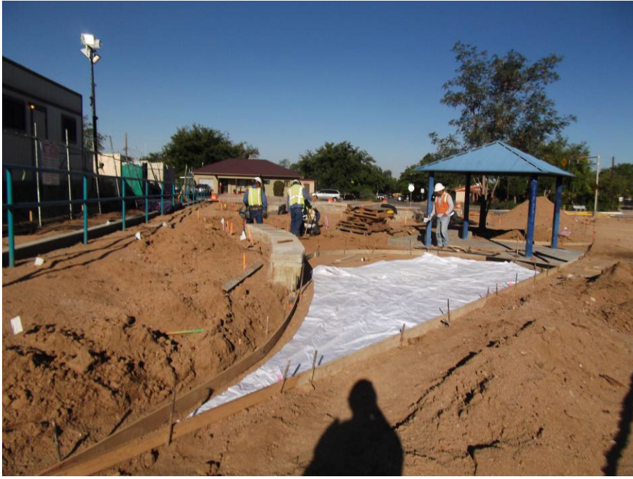
HO Laying out patterns in the pocket park plaza checking dimensions.
