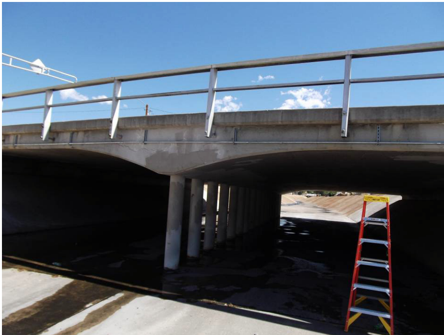
Bixby placing electrical conduit on the west side of the bridge.
