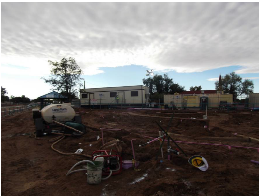
Land Tek pressure testing in the pocket park.
