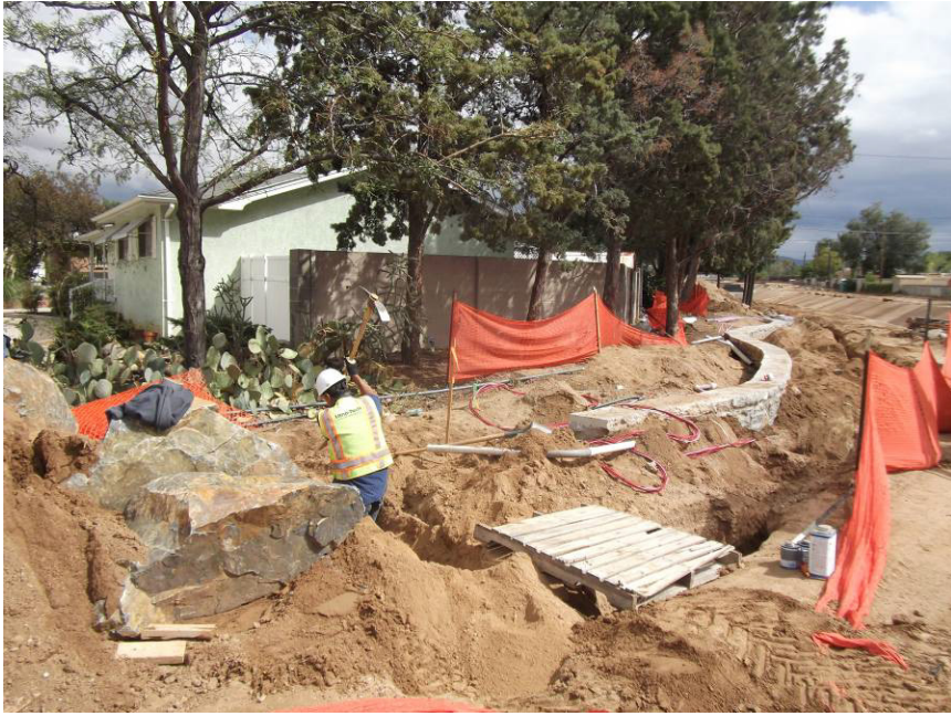
Land Tek trenching to the controller pad.
