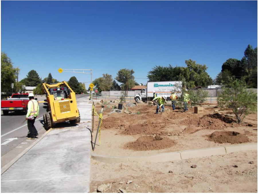
Land Tek placing trees and plants in the pocket park.
