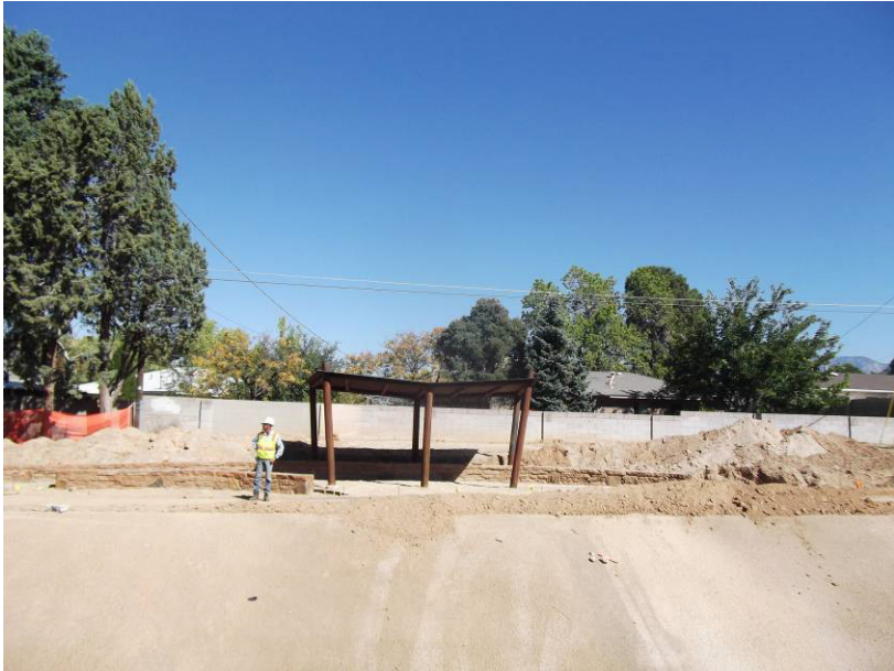
Shade structure – Gallery Paint placed sealant on the structure this morning.
