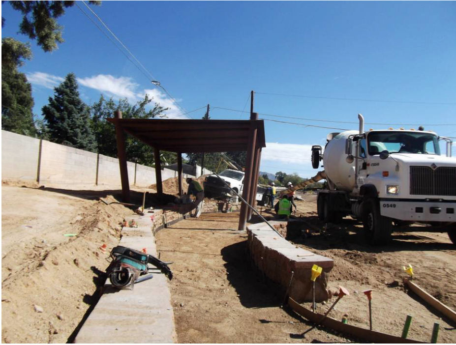
HO placing exposed aggregate under shade structure.
