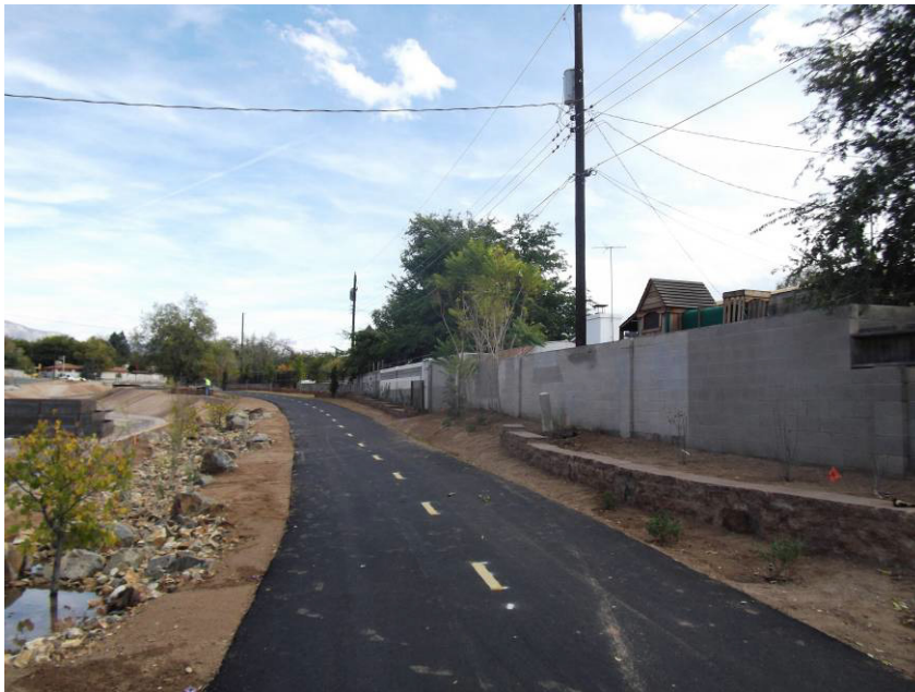
Bike trail on the south side of the channel with striping
