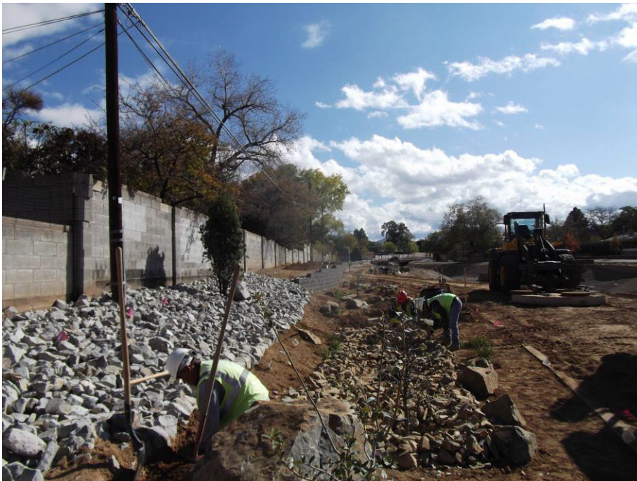
Land Tek working on the north side of the channel.
